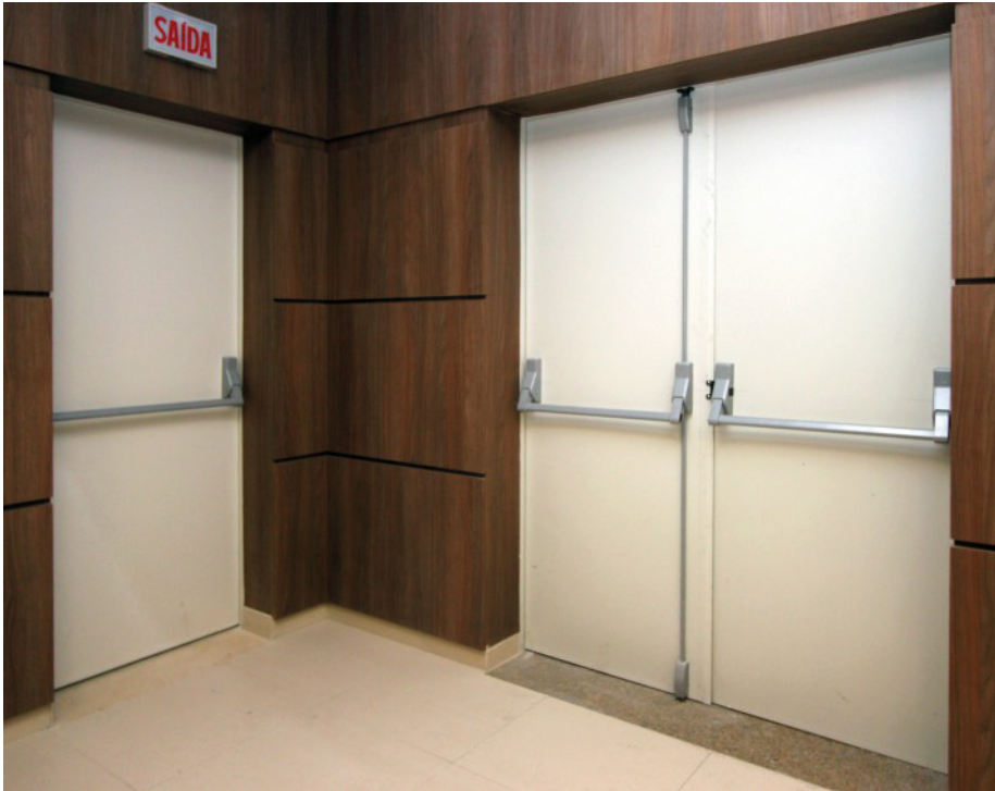
▲ Single leaf door and double leaf door with single and double panic bars
