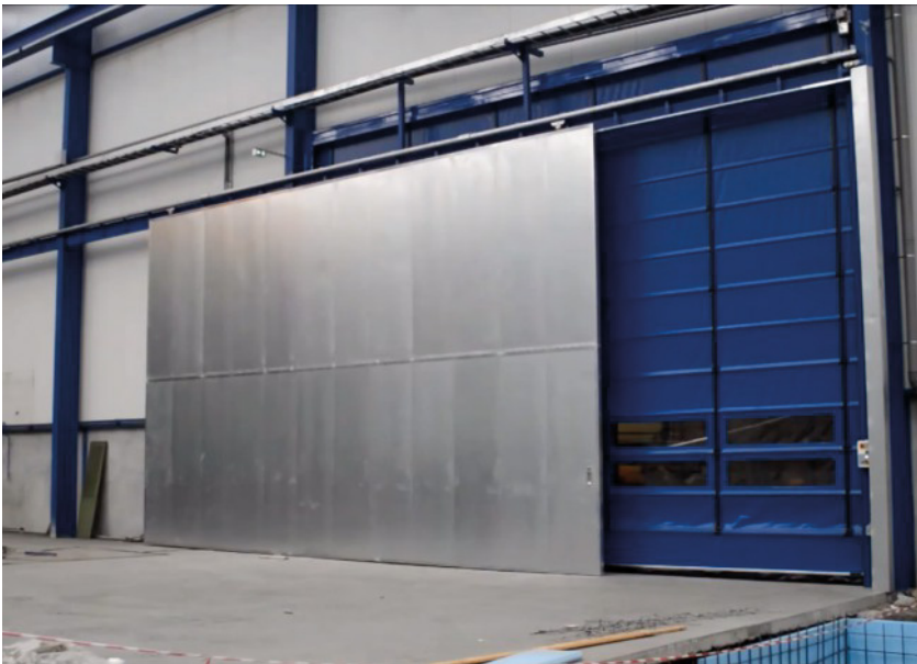
▲ Industrial sliding door with electromagnet closing system and counterweight
